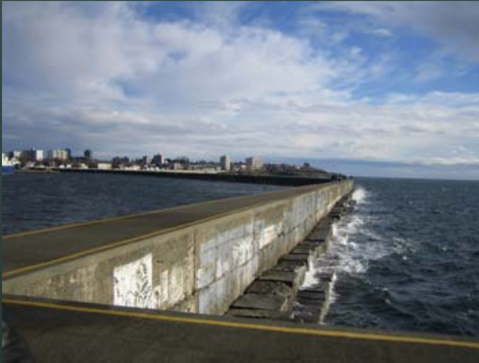
Ogden Point Breakwater Victoria BC
