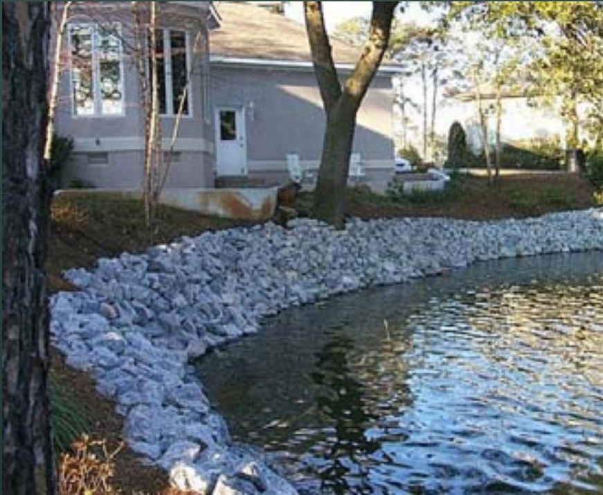
Rip Rap Banks
