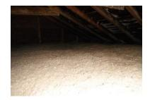
Ventilation: sloped roof: evidence of condensation at underside of sheathing, typically due to inadequate ventilation, provide soffit vents to improve and monitor,
