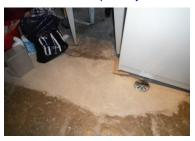
basement rear floor under window: older drain that services exterior walk drain - may require replacement
