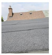
2nd Slope: aging surface, budget to replace within 3 yrs. Garage: overall surface in good repair
