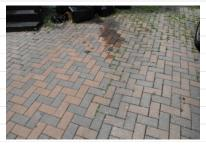
\*\*7.0 Walk(s): seal gaps at wall around perimeter to minimize moisture in basement
