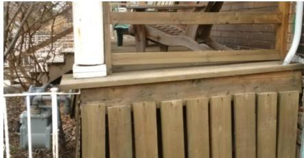
**DECK** overall in good repair, requires safety spindles on rails
