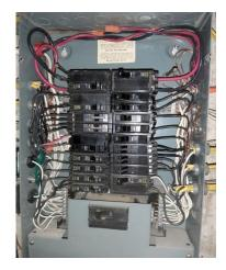
BRANCH WIRING: based on random sampling it was determined the wiring has been upgraded throughout
