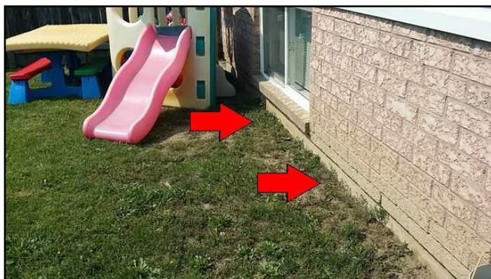
Grading directs water toward Foundation
